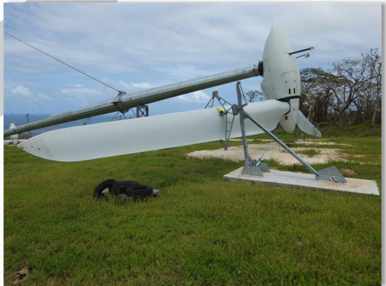
Wind turbine with cyclonic proof equipment on Efate Island
