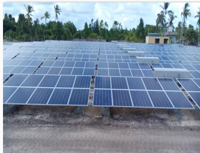
Installation of Vergnet Solar PV panels
