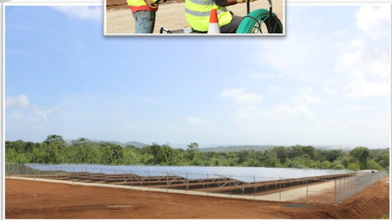
Solution photovoltaïque de Pohnpei - 600 kWc
